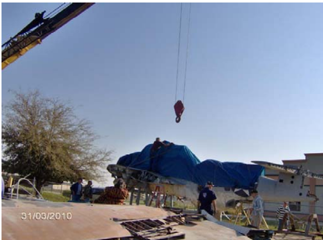
Lowenstein disconnecting rigging to release crane
